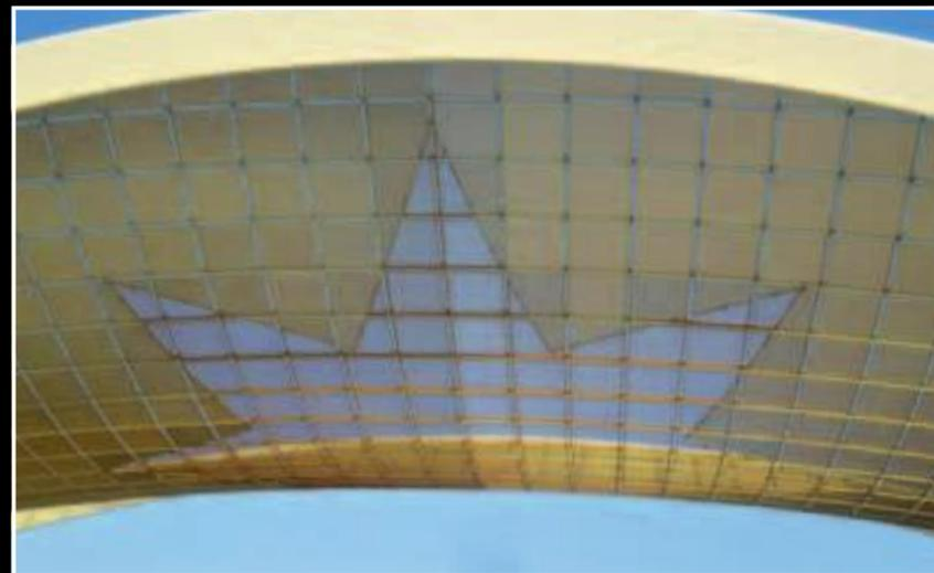
The combination of two meshes with different transparencies enables the star of Azerbaijan to be seen. On the inside of the star the texture of the mesh is Coliseum in a darker golden anodised colour while on the outside the mesh is Academy in a lighter shade of gold.
